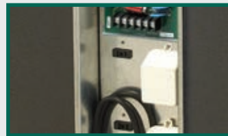
Electrical Compartment for 4 Accessory Transformers, and Mounting Space for Surge Suppressors and an Access Control Radio Receiver
